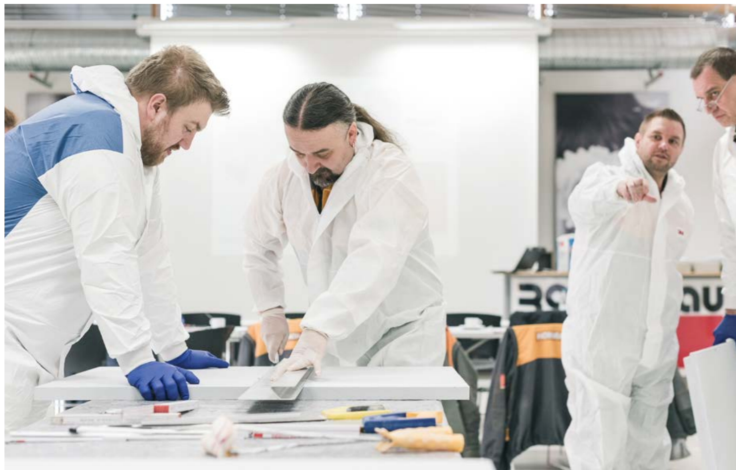
Trimming the calcium silicate board (above) is new to many participants, but actually surprisingly easy. As well as numerous practical exercises, the training also includes a theory module (right)
